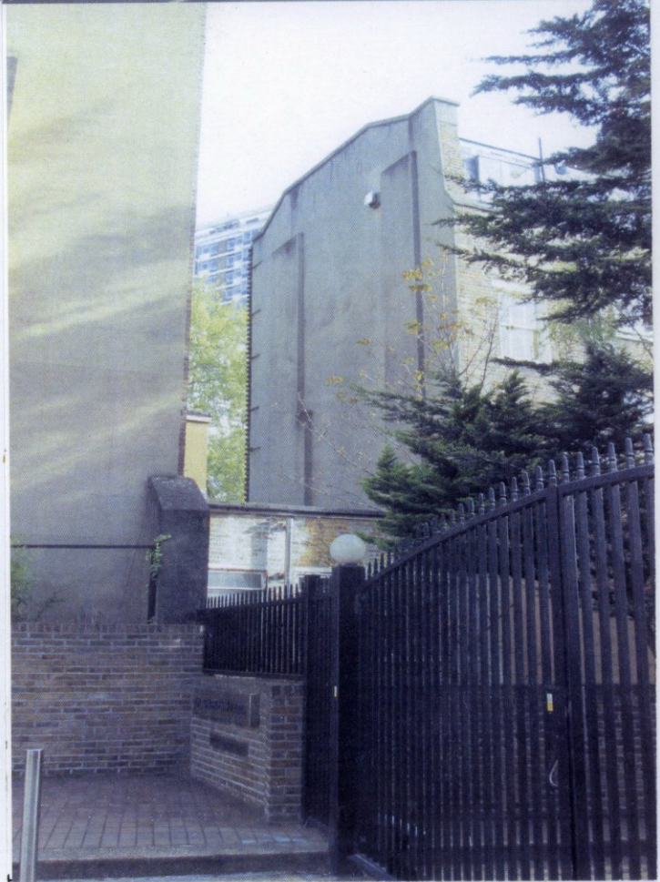
59 Connaught Street front elevation looking west (top) and rear elevation taken from Albion Street (bottom)
